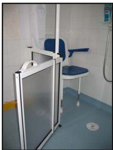
Wet room former with waterproof floor covering
